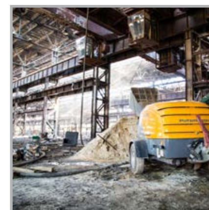
Russia, Ryazan placement of ~ 100,000 m 2 of screed
