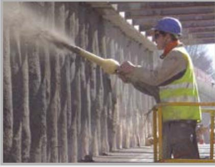
Fine concrete pumps like the P 715 are among the most versatile systems. You can use them for shotcrete or for pumping fine concrete with a grain size of up to 16 mm.
