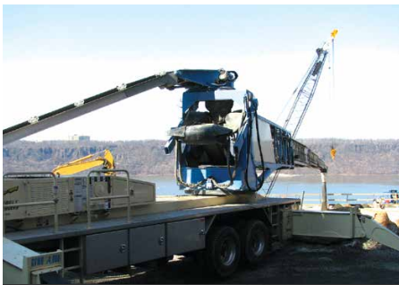
A CLEAN, EFFICIENT & LOWER COST SITE
