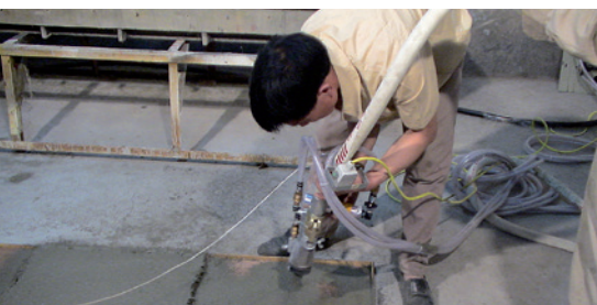
MAKING FIBRE-REINFORCED CONCRETE SLABS
