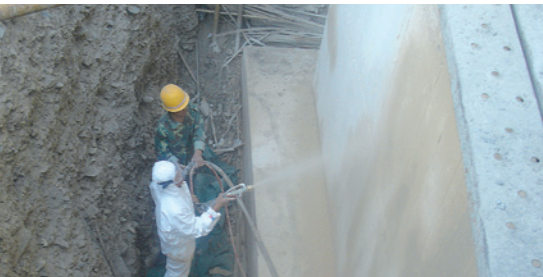
COATING CONCRETE FOUNDATIONS
