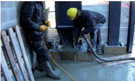
FILLING STEEL COLUMNS
