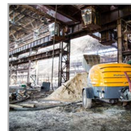
Russia, Ryazan placement of ~ 100,000 m 2 of screed
