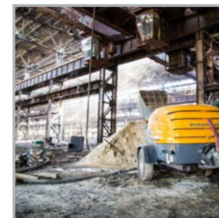
Russia, Ryazan placement of ~ 100,000 m 2 of screed
